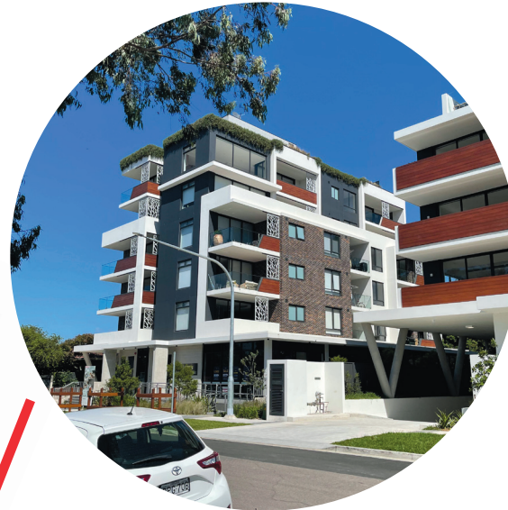
EXISTING CONDITION ON HINKLER AVENUE
